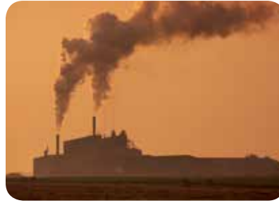
Industries, HVAC & Marine
